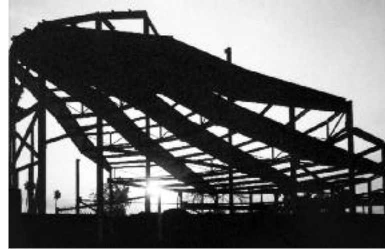
As the girders were raised, it was noticed that skeletal structure of Shumei Hall resembled a human hand, outstretched as if to give a blessing.
